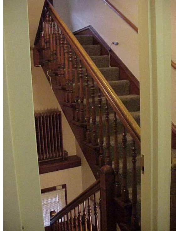
Figure 5.13 First Floor Leading to Basement
